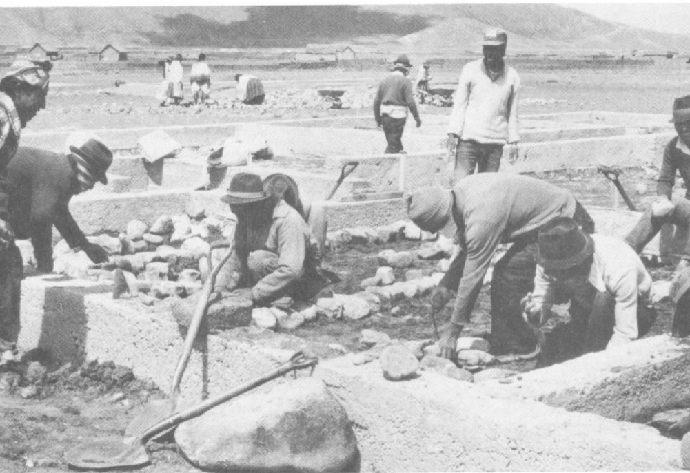
Labor marchers in La Paz Building a sheep-breeding facility at Lake Titicaca Courtesy Inter-American Foundation (Kevin Healy)
